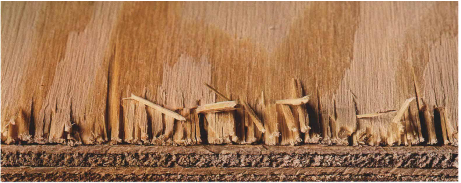
The ragged edge. A circular saw left a trail of destruction across the grain of this ½-in. AC plywood. This could easily have been prevented.
